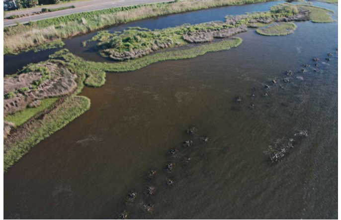
This photo shows the layout of the Project Greenshores living shoreline. The breakwaters are visible along the marsh edge. These structures help to reduce wave action.
